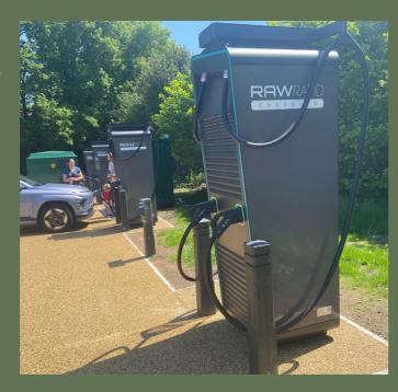
EV Charging - HoT Mill Meadows Car Park, RG9 1BE, 2 x Type 2 (22kW), 2 x CCS (up to 50kW) Mer charging units.
